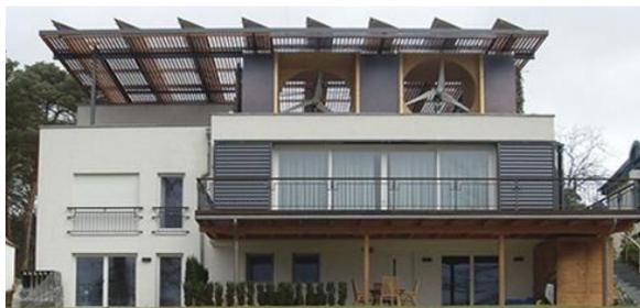
*Fig. 9: test and reference building implementing in-house micro-wind-turbines, PV, CO<sub>2</sub>-heat-pump and 12m<sup>3</sup> heat storage and management system*
