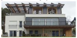
Fig. 9: test and reference building implementing inhouse micro-wind-turbines, PV, CO<sub>2</sub>-heat-pump and 12m<sup>3</sup> heat storage and management system
